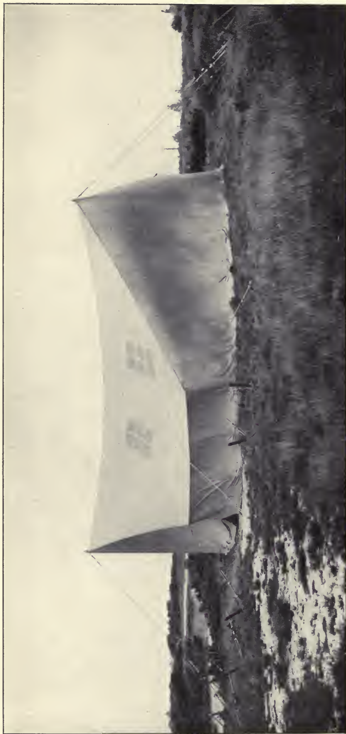
FIELD TENT FOR AEROPLANE: BACK VIEW. Supported by two poles only; Roof ridge formed by stretched wire rope. Designed R.A.F. 1913.
